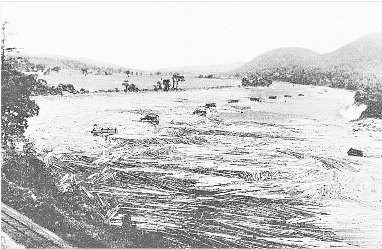
This historic photo shows logs in the Connecticut River in Bellows Falls. The piers were used to anchor the chains and cables that created large, individual corrals in the river for lumberjacks to organize the logs.
