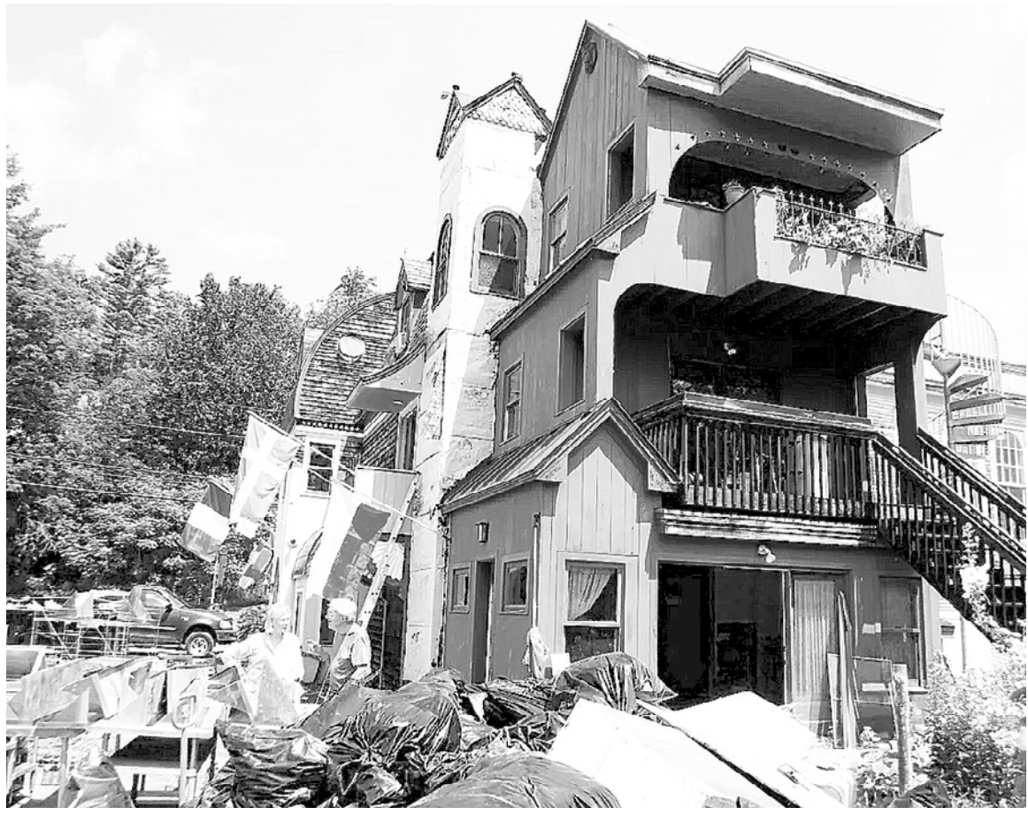
Judith and Tom Platt assess recent flood damage to their Garden Market, Café and Gallery in Londonderry.
