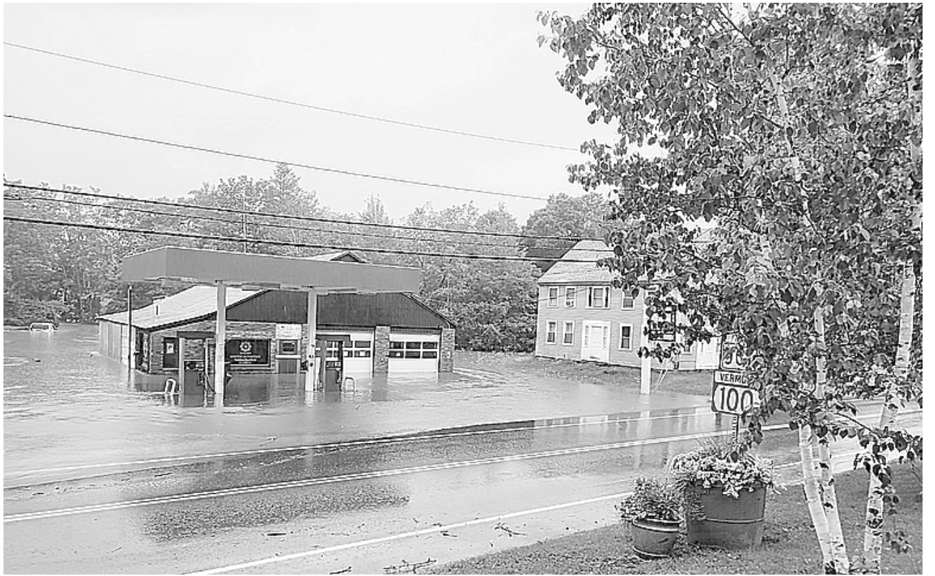
Green Mountain Therapeutics in Londonderry was just weeks away from opening when the West River overflowed its banks on July 10 and flooded the building. ERIC SCHWIPPET/SPECIAL TO THE COMMONS
