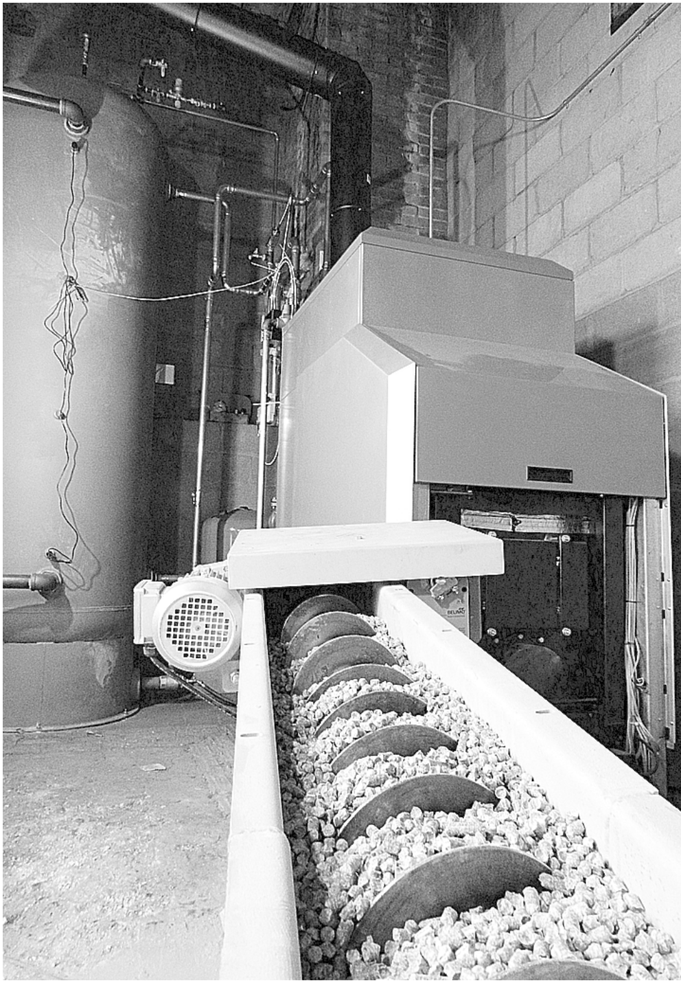
Wood pellets are fed into the EvoWorld boiler at the Vermont Farmer's Food Center in Rutland.
