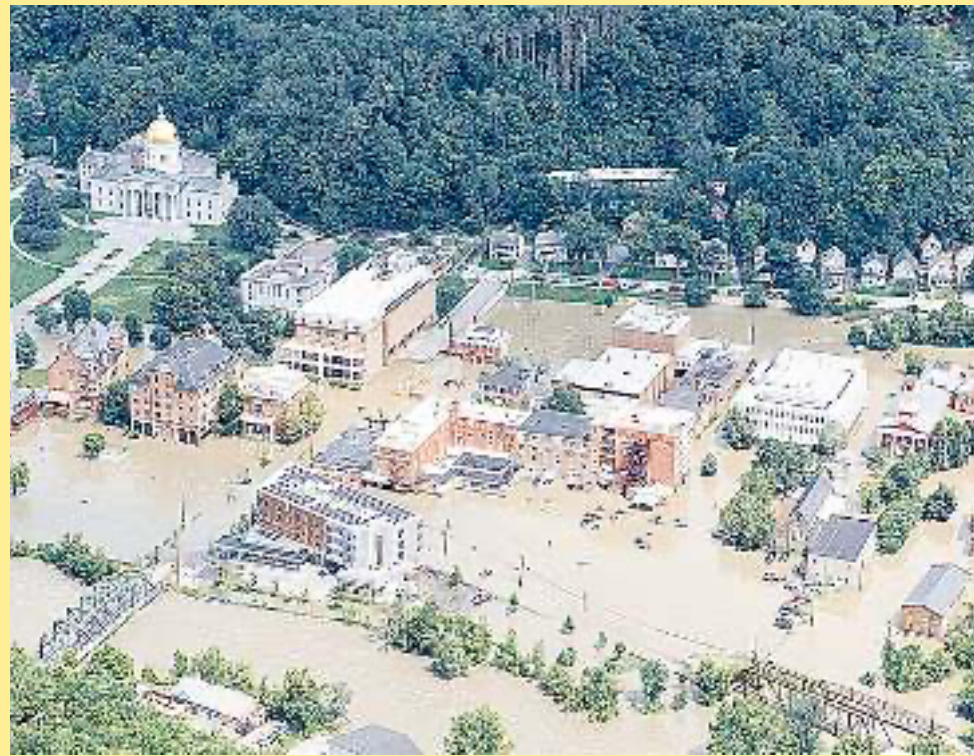
Downtown Montpelier under water on July 11 following record heavy rains.
