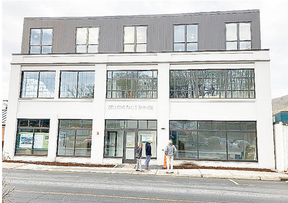
While the original Bellows Falls Garage needed to be demolished, its concrete facade was recreated in the new structure.
